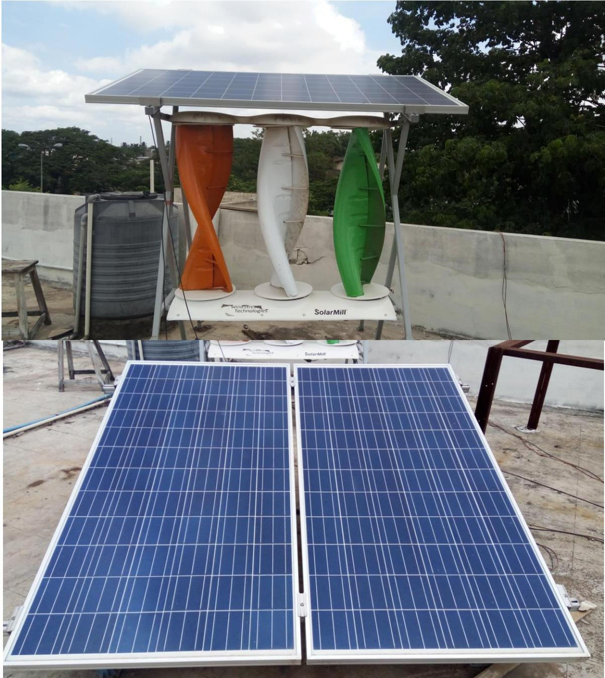
**Photo 4- Hybrid solar and wind power plant.**
