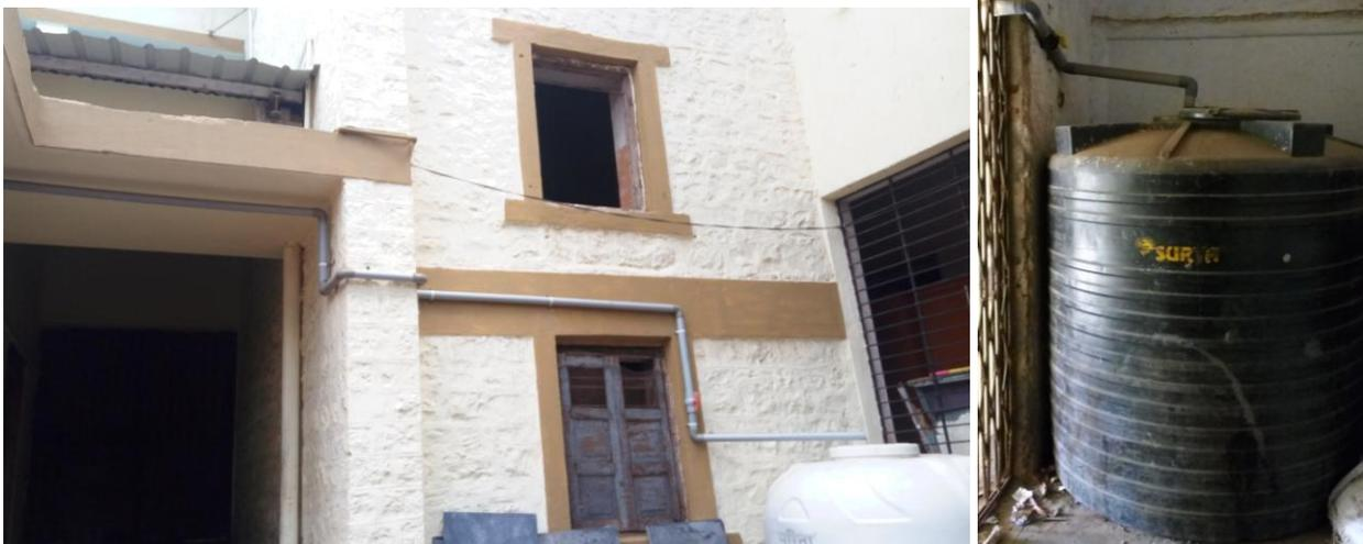
**Photo 6-RWH system provided with centralized storage tanks.**
